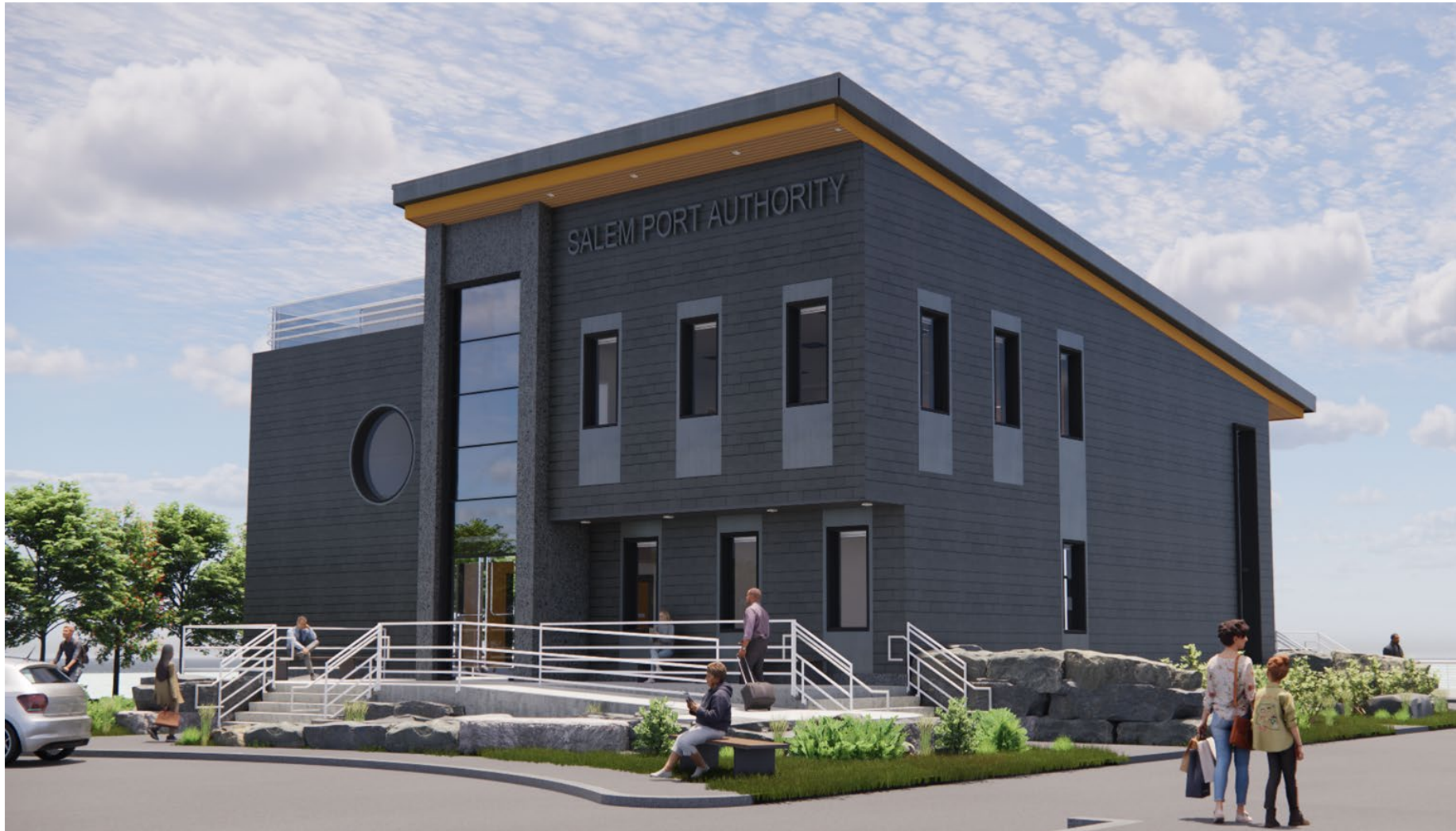
BUILDING EXTERIOR FROM LANDSIDE
